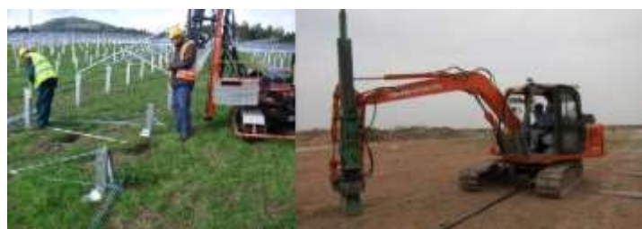
Figure 11: Installation of frame foundation (Image from www.aceinfra.com and www.kaska.eu )
