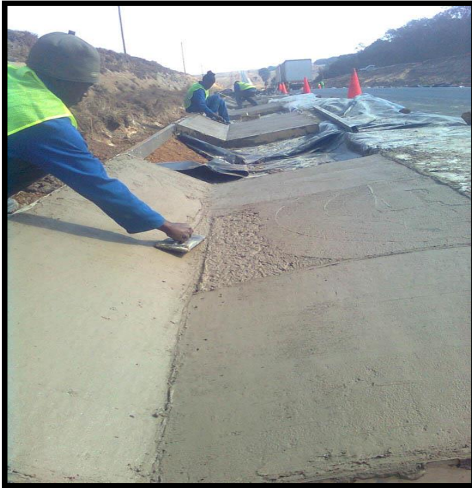
Photograph 2: Showing the construction method of the proposed V-drains.
