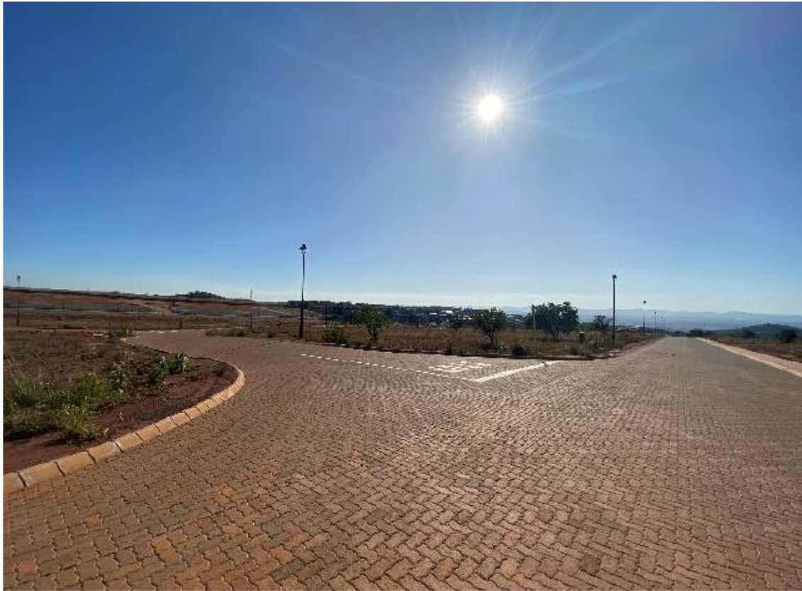
Figure 7: Recently paved roads forming part of an adjacent approved development.
