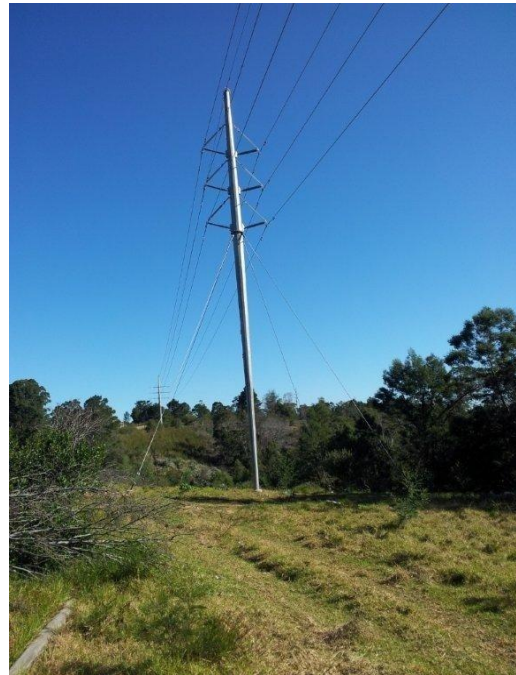
Figure 2.3: A guyed intermediate post. Source Aurecon
