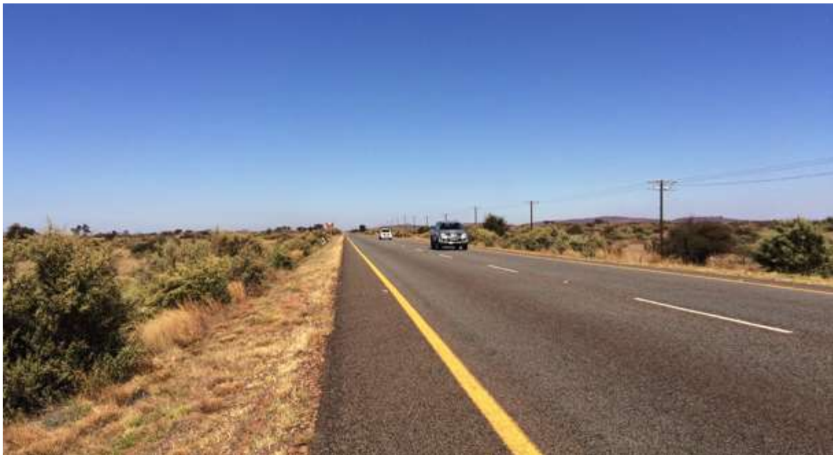
Figure 5: Photograph taken in a southerly direction of the N14 National Road.
