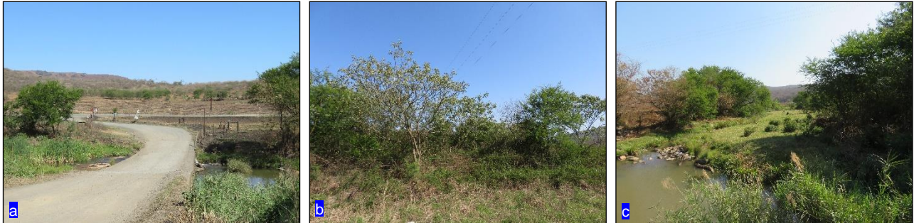
Figure 5: (a): The current crossing, facing east. (b): The vegetation on the western bank of the river. A mix of indigenous and alien species. (c): A view of the proposed bridge site from the existing crossing structure, facing south.
