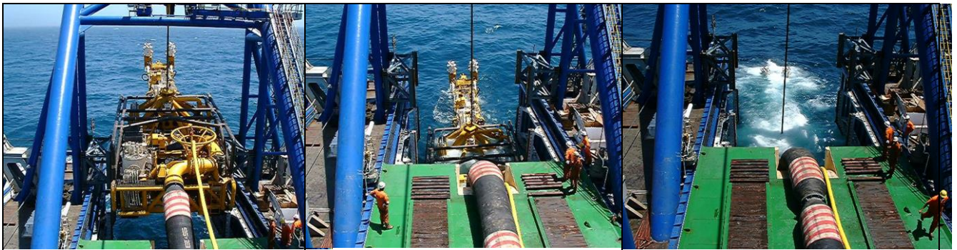
Figure 4-3: Deployment of the seabed crawler
