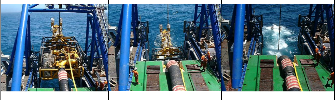
FIGURE 3-2: DEPLOYMENT OF THE SEABED CRAWLER
