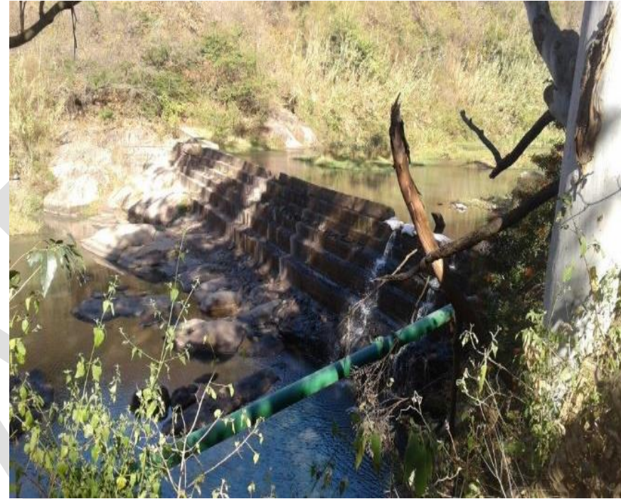
Photo 8: View from the left hand bank of the Umzinto River looking from north to south across the river showing the proposed site of the new gauging weir which will be mounted on the existing infrastructure.
