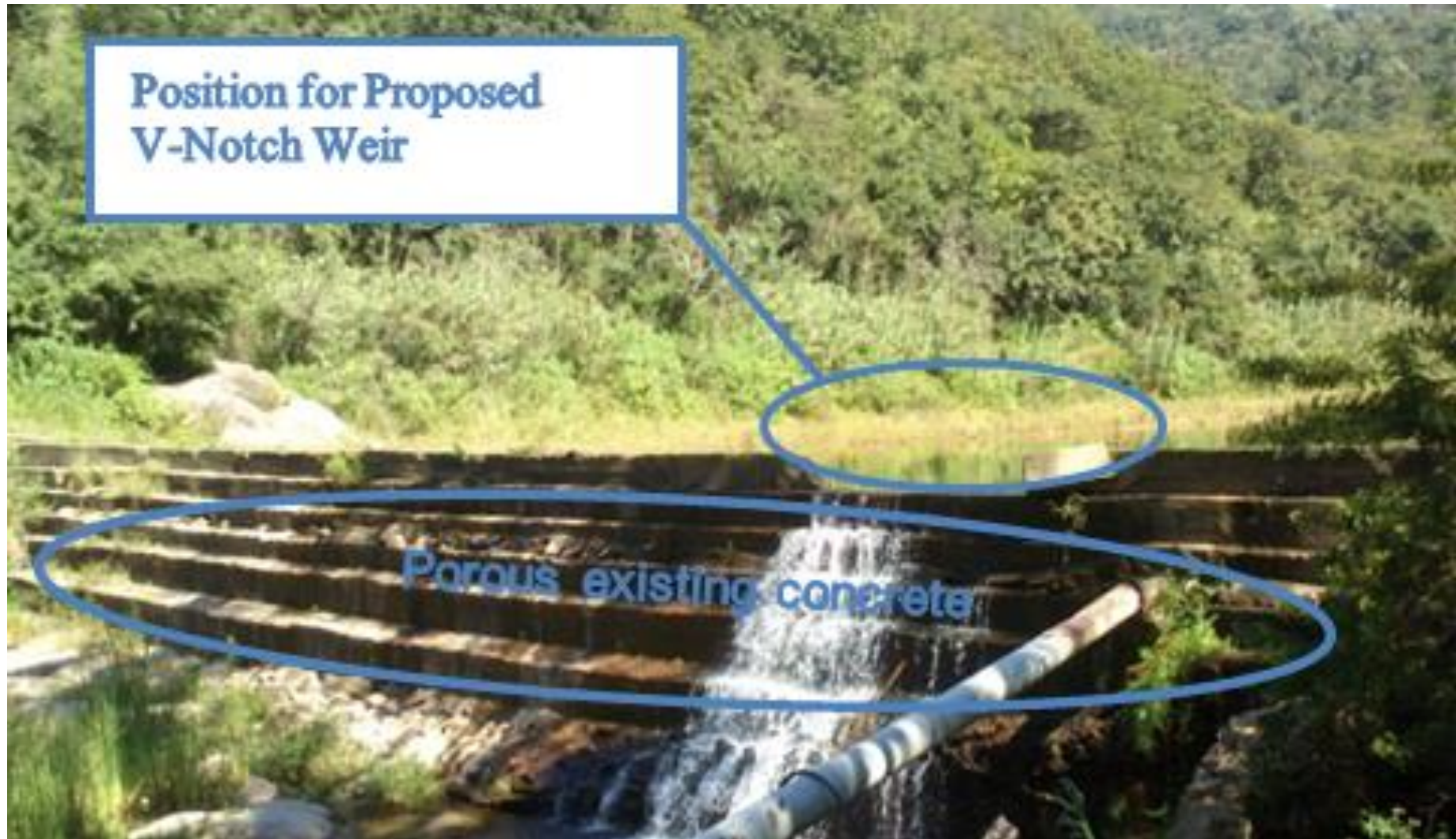
Figure 4: Position for the Proposed V-Notch Weir
