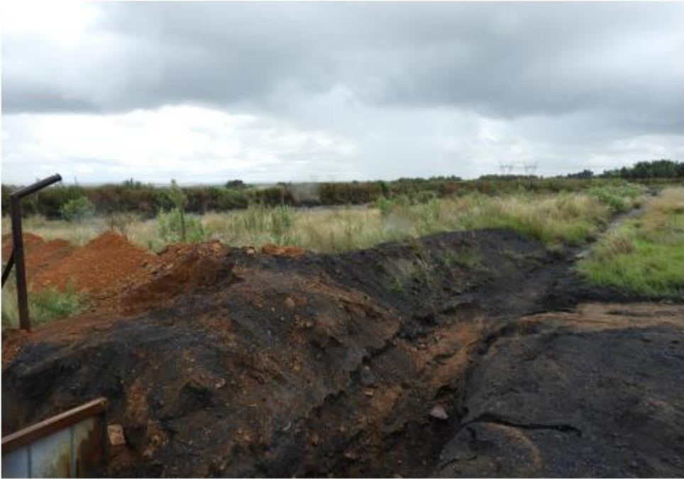
Photograph 3: Channels dug around the site leading to the "sludge area"
