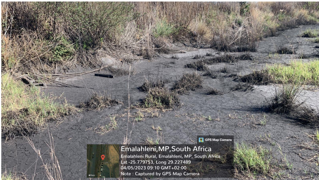
Figure 6: Evidence of a coal sludge at the processing plant area.
