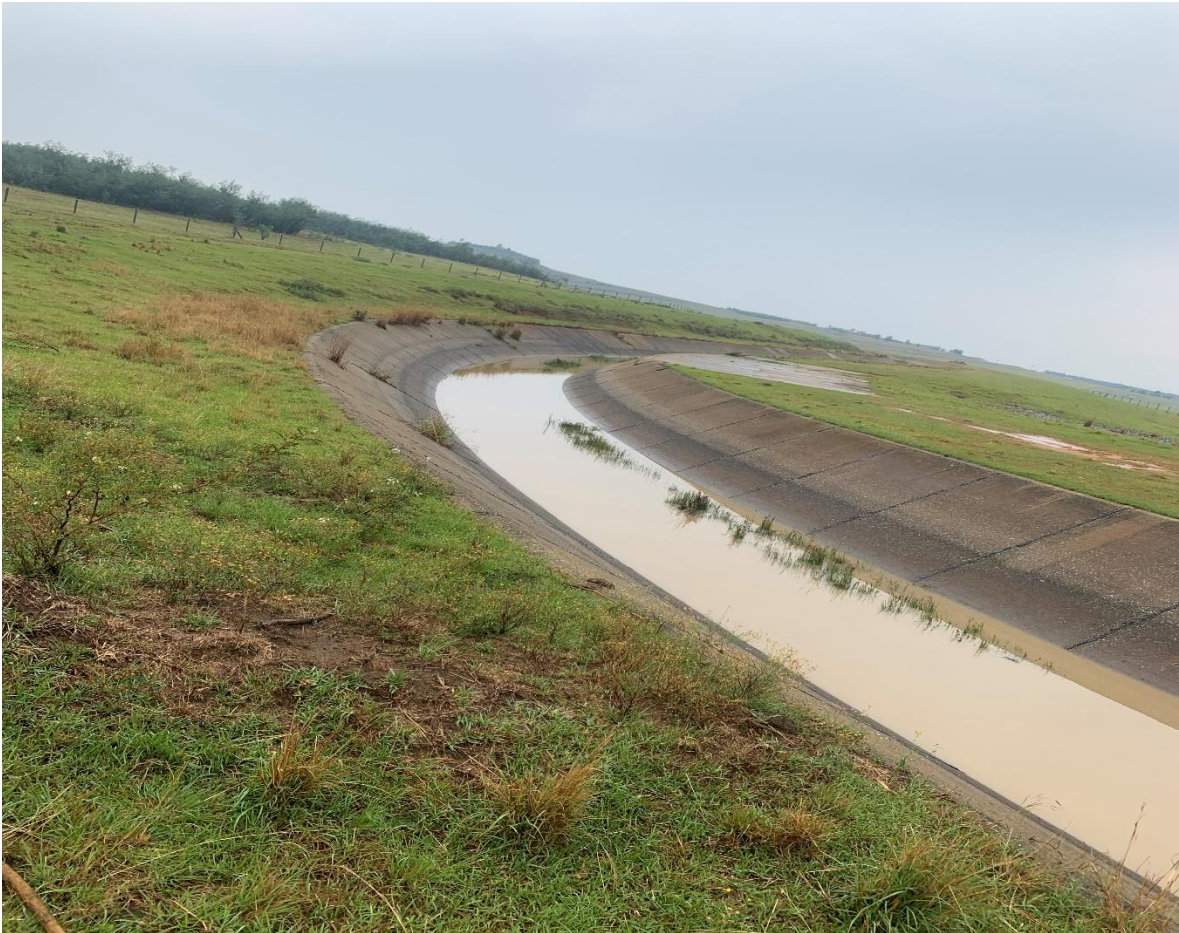
Figure 25: Dirty water trench on-site (Site Visit, 2022)
