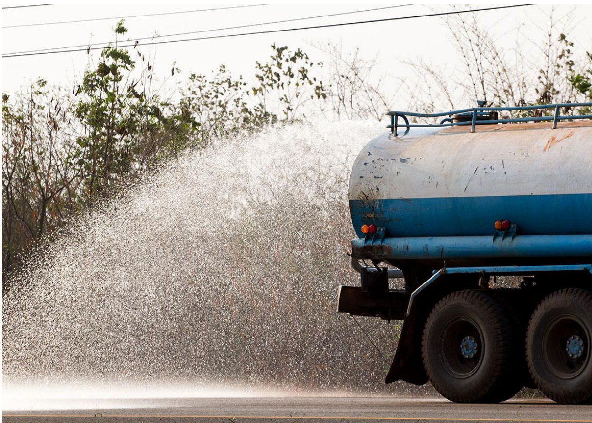
Figure 37: Example of a dust suppression (water spraying)
