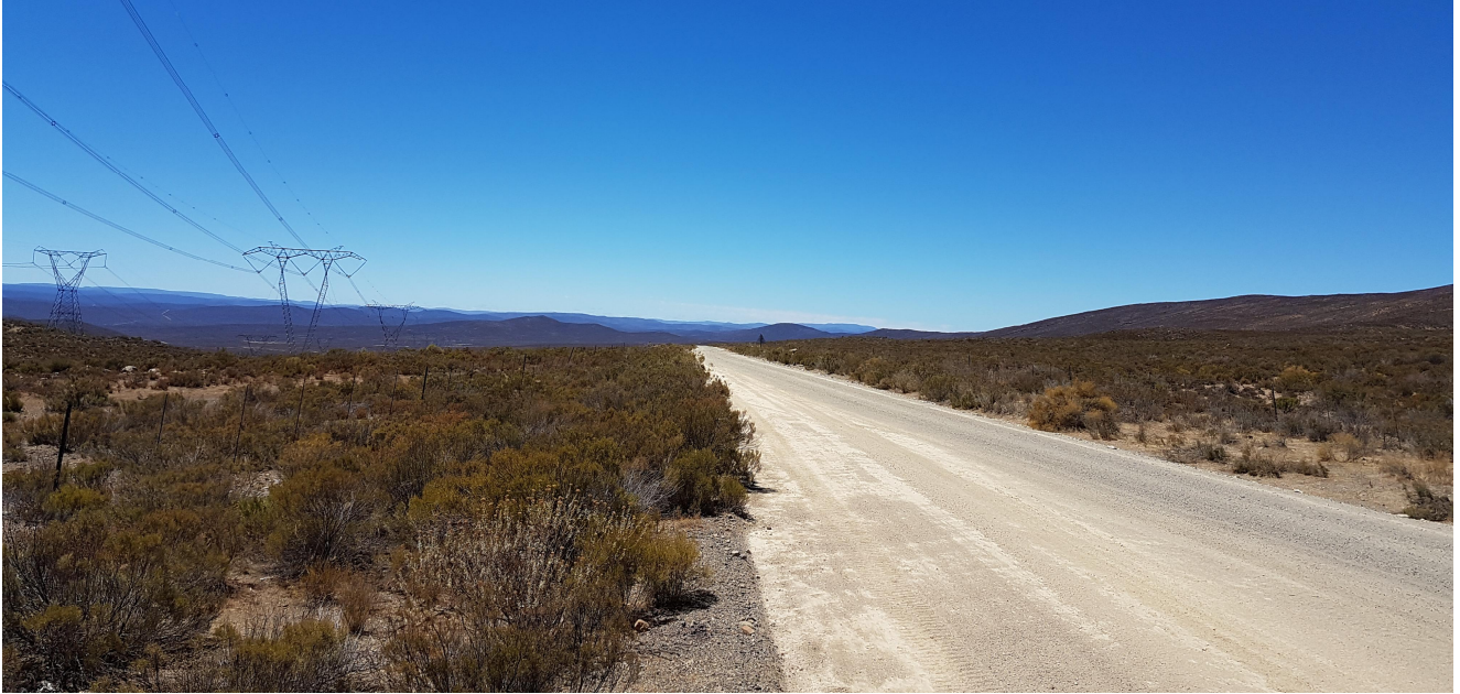
Photograph 3: The existing road and Eskom Powerlines, which run adjacent to the proposed Esizayo Powerlines to the Komsberg Substation.
