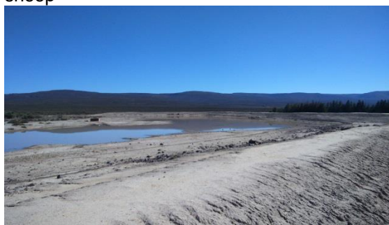
Plate 4: Earth-wall dam with water
