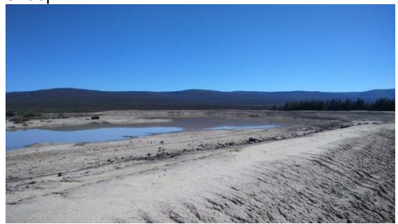
Plate 4: Earth-wall dam with water
