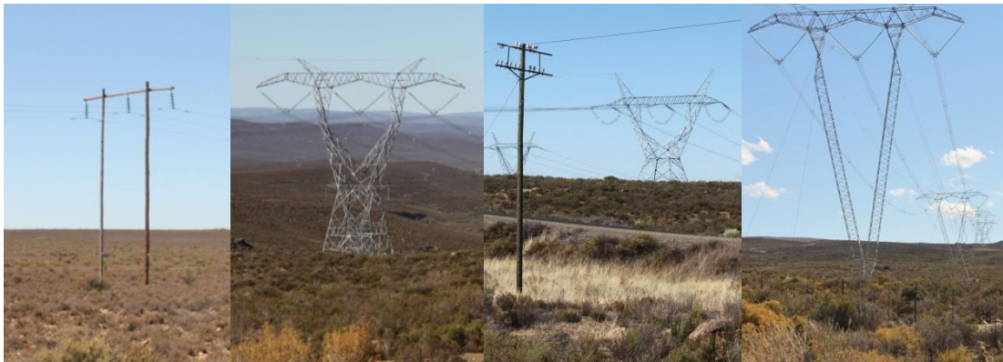
Plate ix: Existing power towers in the vicinity
