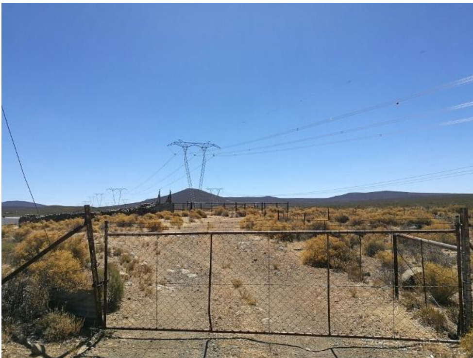
Figure 13: Power pylons near the R354
