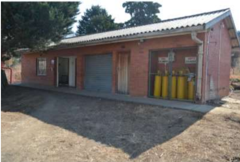
Figure 15: Existing treatment works building
