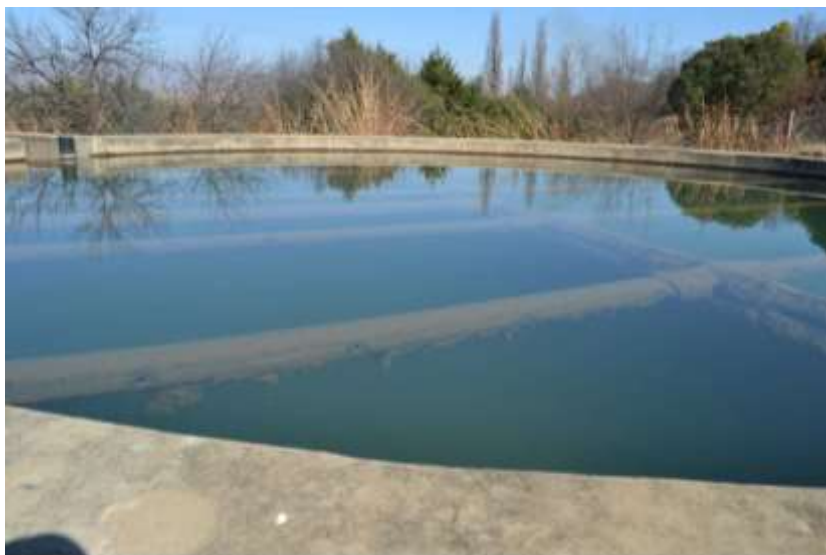
Figure 8: Launder pipes installed within clarifier
