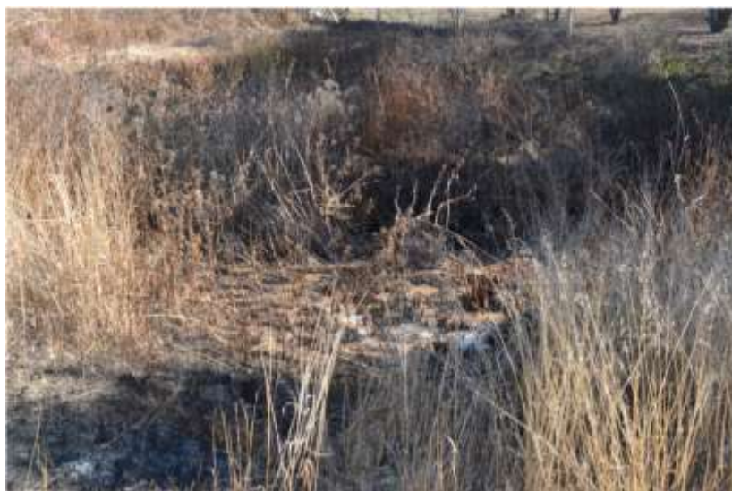
Figure 10: Sludge drying bed
