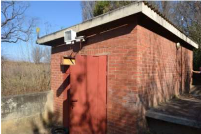
Figure 1: External view of raw water pump station
