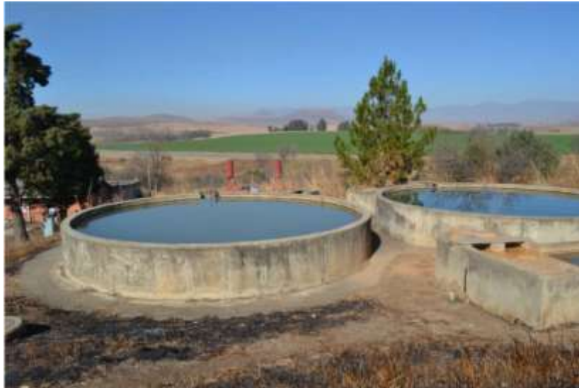
Figure 7: Circular sedimentation tanks
