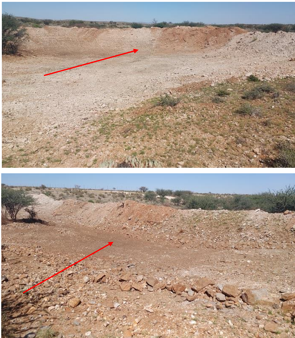
Figure 5: Two images illustrating examples of the ten small artificial earth dam walls that have been constructed within the various watercourses and which are significantly impeding the ephemeral flow regimes of the watercourses (red arrows indicate the water flow directions)
