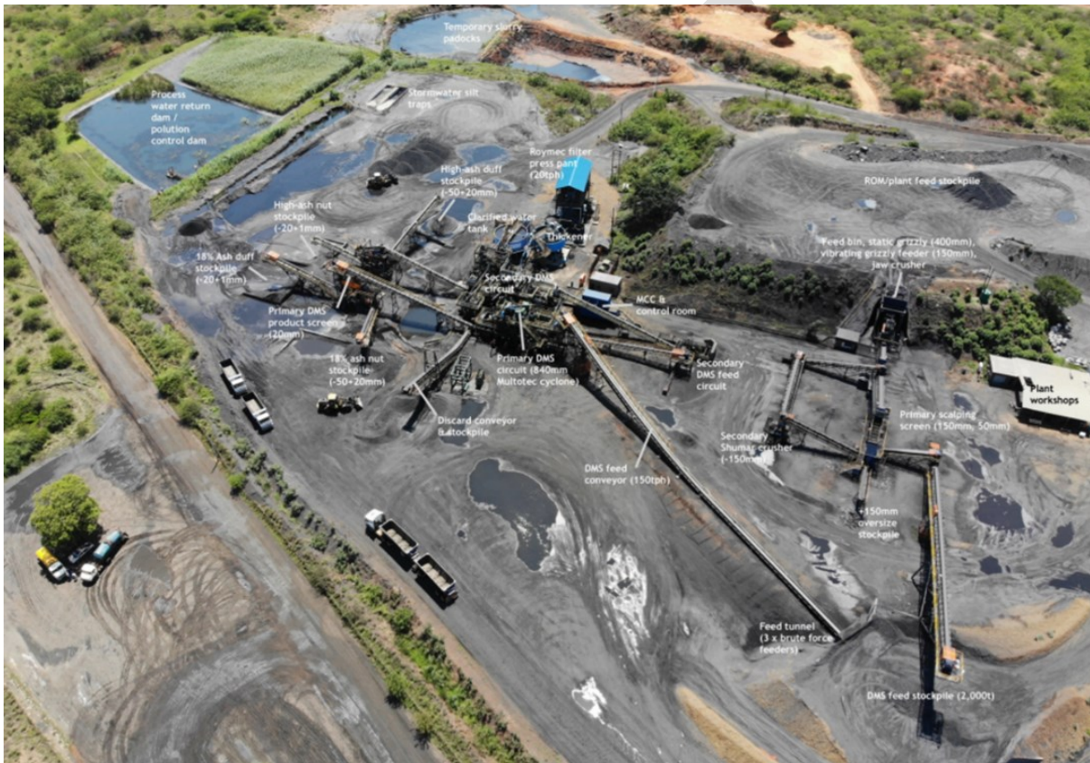
Figure 4-4: Photograph of Processing Plant
