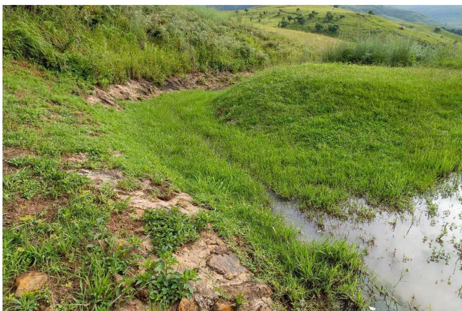
Figure 6. Boma dam spillway (Robinson, 2021)
