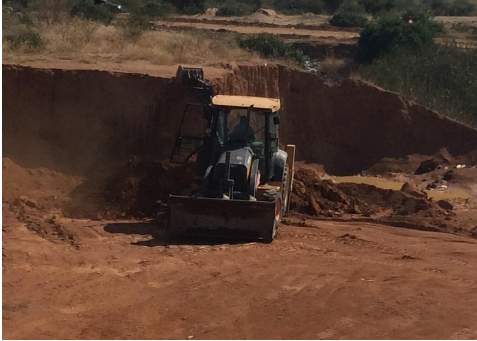
Figure 19: Excavator operating on neighbouring borrow pit site
