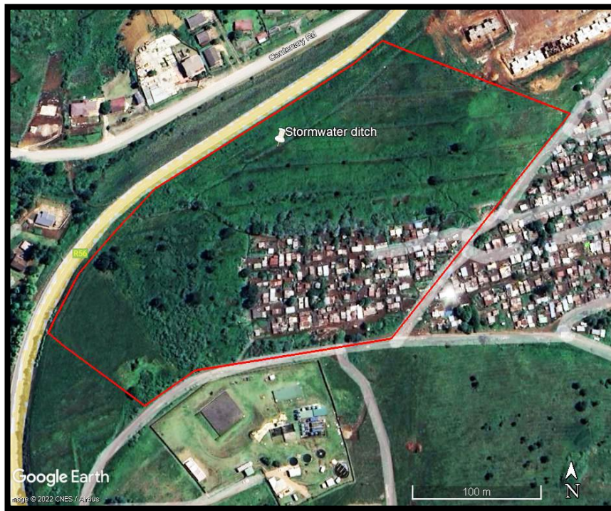
Figure 12 Indication of ditch that serves as stormwater canal at present.
