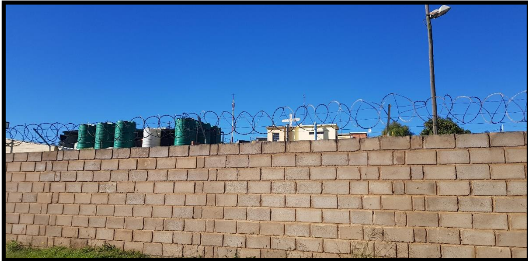
Photograph 2: The site is bordered by the Ixopo water treatment plant towards the South
