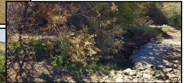
Photo 3: Northern side of the watercourse crossing
