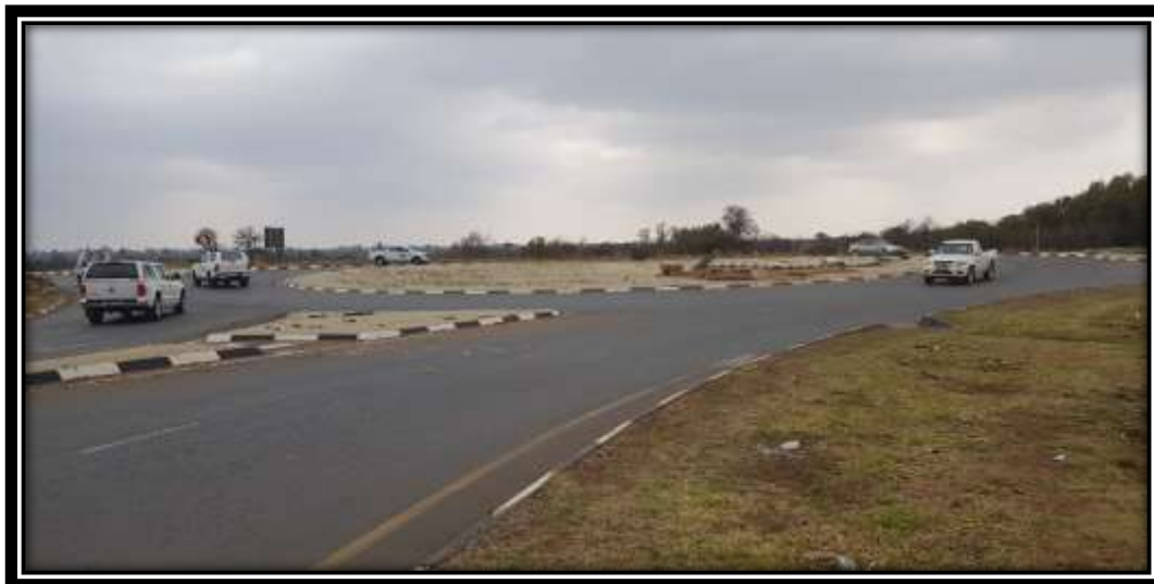
Photograph 2: The newly constructed traffic circle
