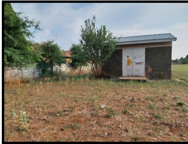
Photograph 3: There is an electrical substation on site
