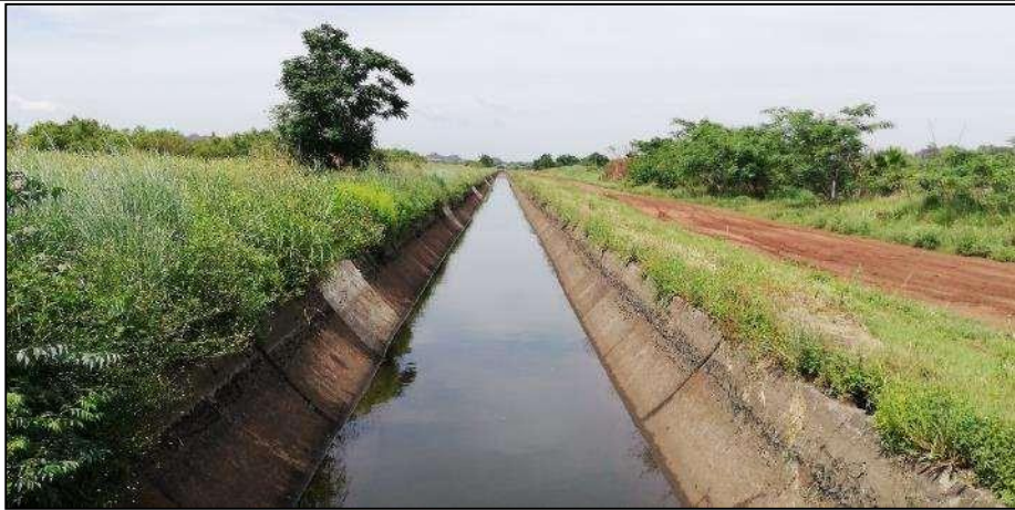
Figure 24: Canal associated with RE/14/420.
