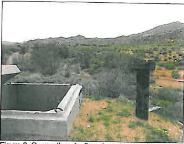
Figure 9. Connecting pipeline alongside the N7
