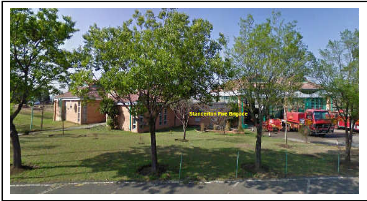
Figure 13: Standerton Fire Brigade
