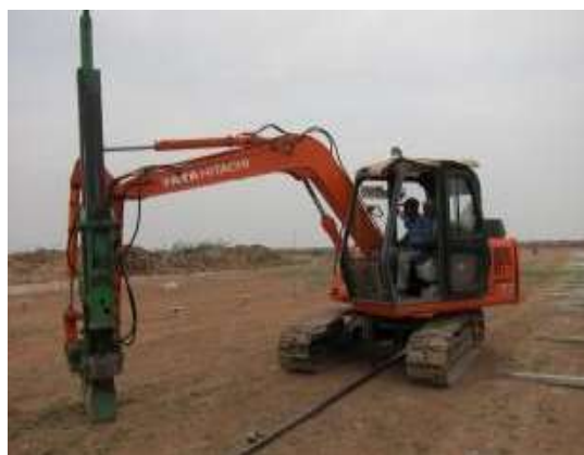
Figure 2.2.: Installation of Rammed Pier foundations
