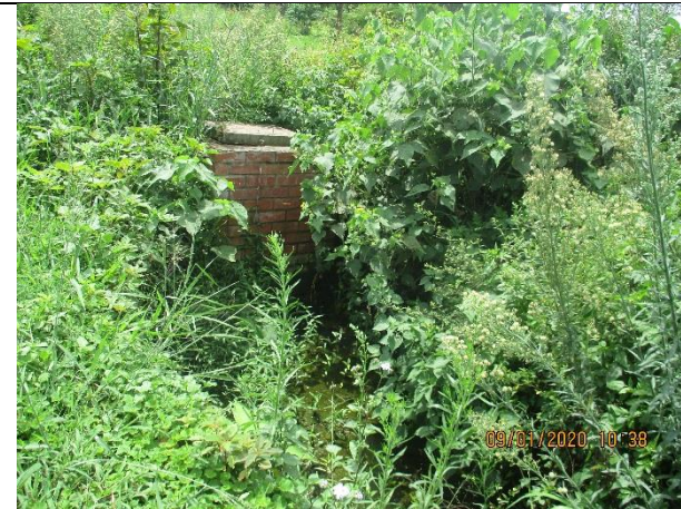
Photograph 8 : View of structures observed on site.
