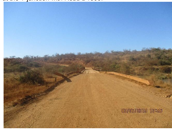
Photo 4: View of the existing single lane bridge over the Mozana River crossing point.
