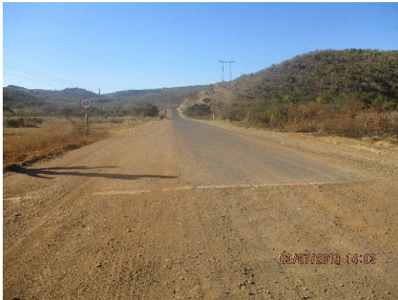
Photo 1: View of the Start point of Road D1867 from Km 6+000 where the Phase 1 of the project ends.
