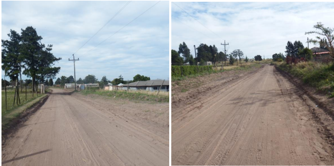
Figure 4-3: Views of the ND500 alternative route along internal gravel road
