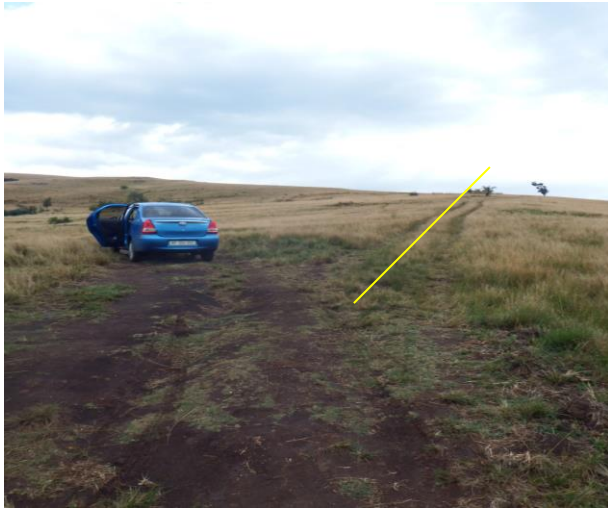
Figure 4-8: View along the secondary road towards the new reservoir R1-2 site
