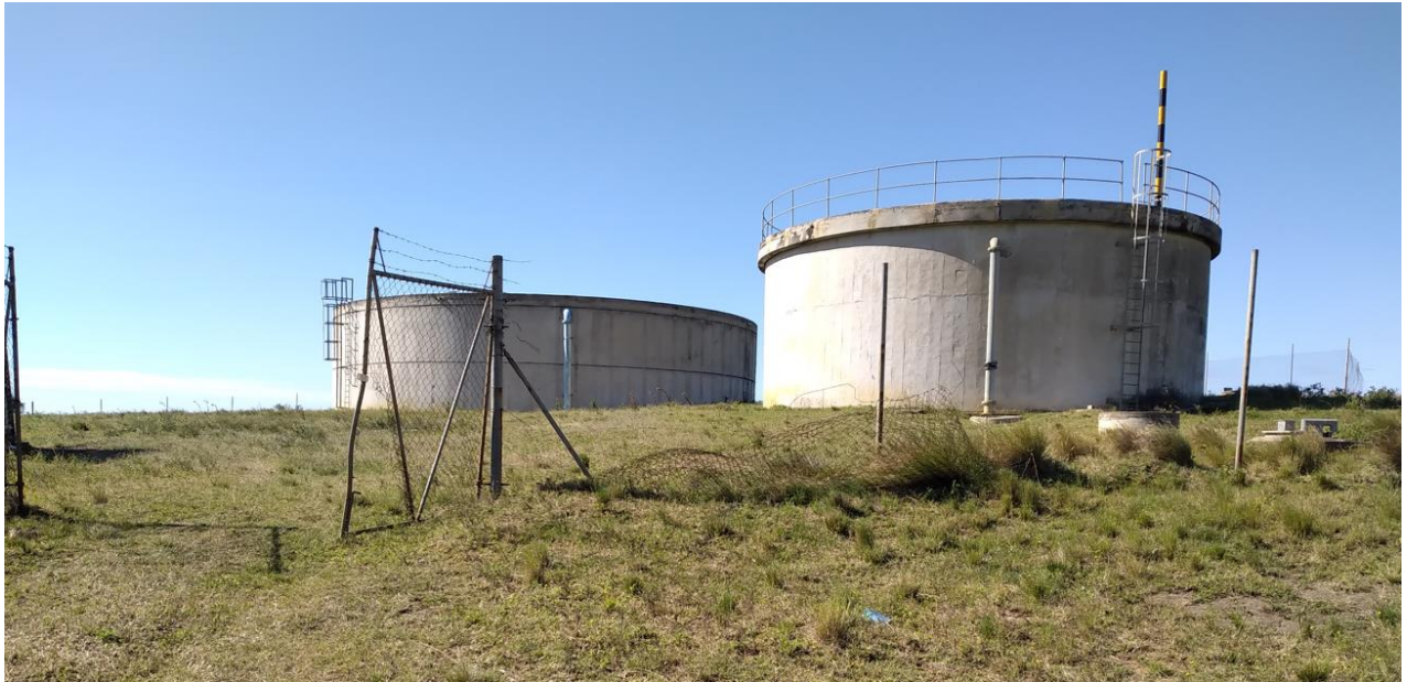
Figure 4-14: Existing Reservoir (R 2-1)
