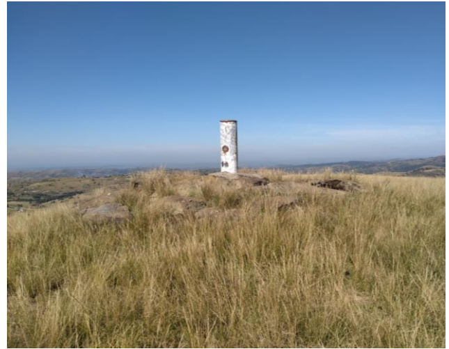
Figure 4-9: Trig Beacon at new reservoir site
