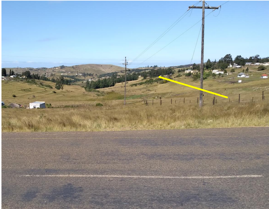
Figure 4-6: View from P230 towards new reservoir (R1-2)
