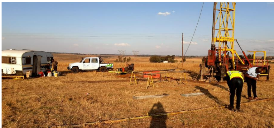
Figure 4: A typical example of diamond core drilling rig.
