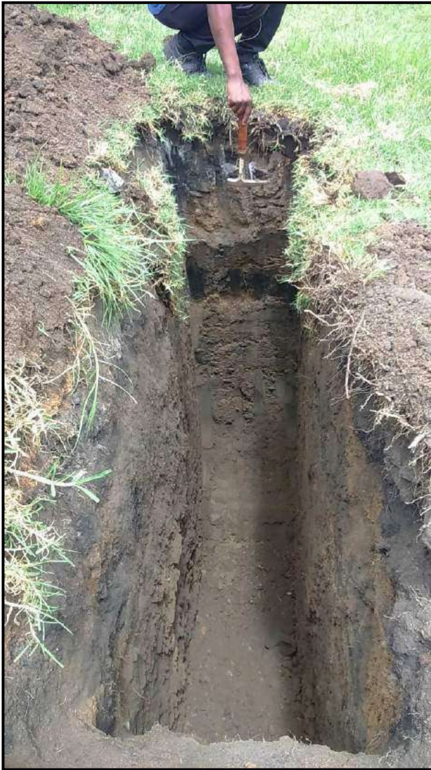
Figure 5 Picture showing typical trial pit along the reticulation pipe network
