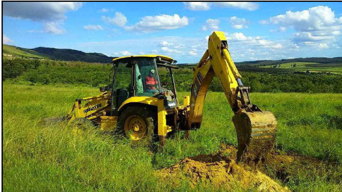
Figure 4 Picture showing trial pit excavation on site
