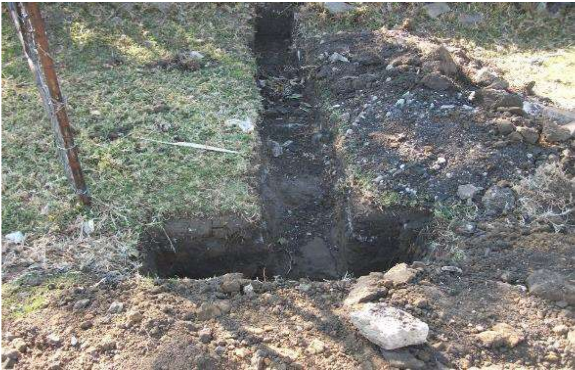
Figure 5: Dug section entering property from road
