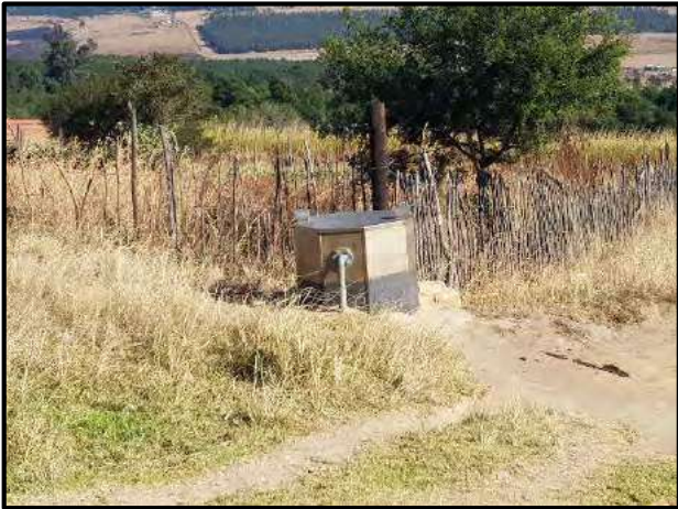
Plate 3 – View of Water Manhole
