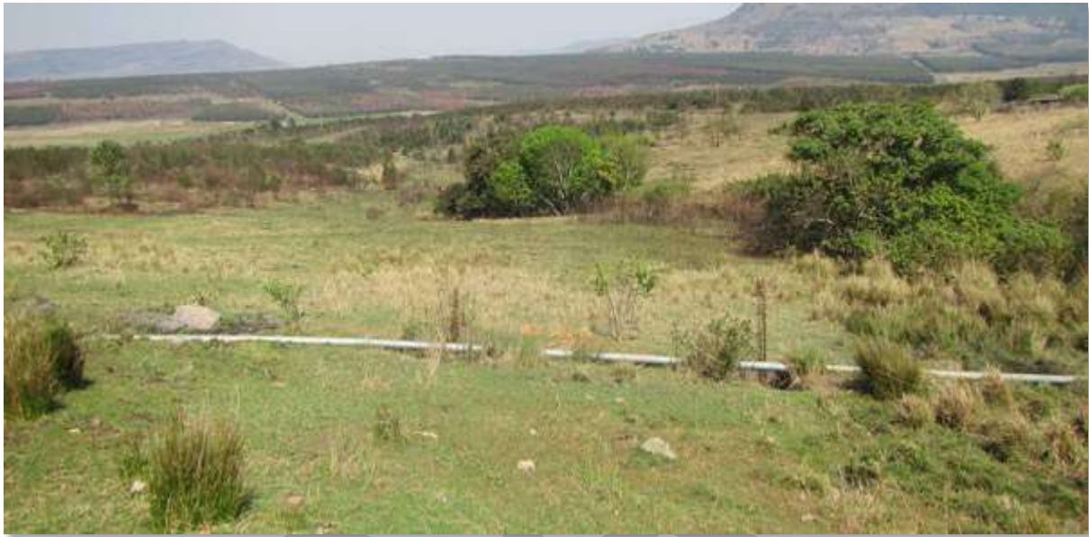
Photograph 3: Drainage channel noted on the north eastern boundary. Note the pipeline already traversing the channel from the previous contractor.
