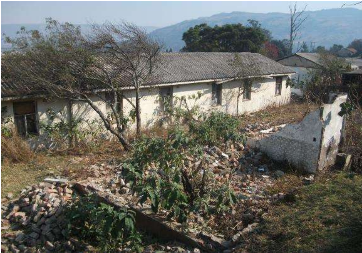
Figure 9: Section of intact compound and remains of demolished section
