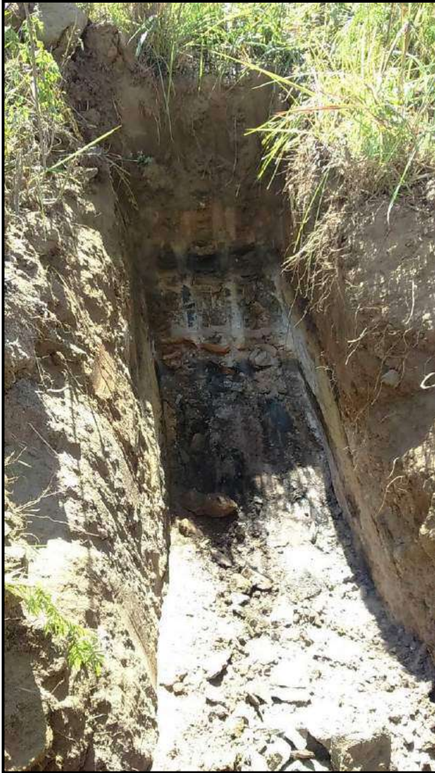
Figure 6 Picture showing shallow sandstone refusal at TP10
