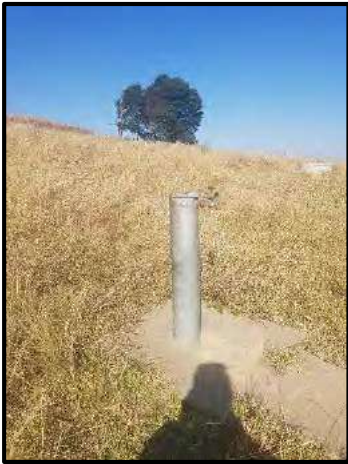
Plate 7 – View of Existing Tap
