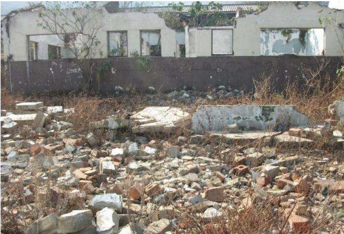
Figure 8: Remains of compound
