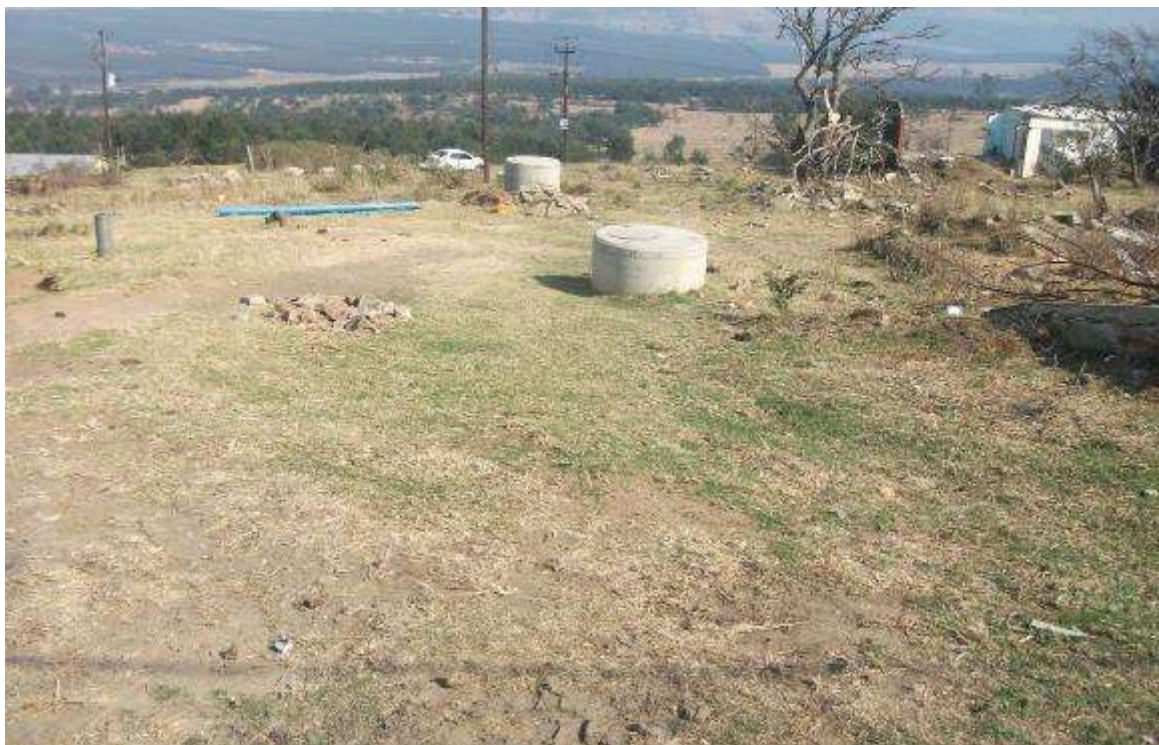
Figure 11: View of pipeline route showing new man-holes
