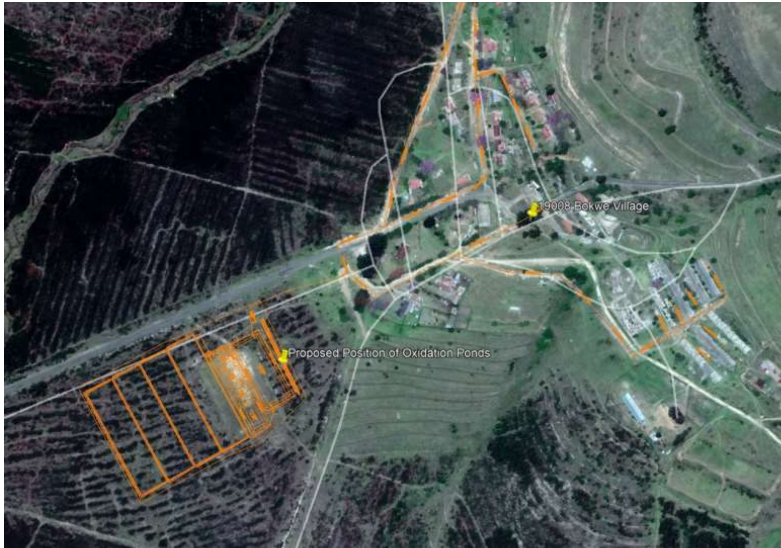
Figure 3: Project layout indicated in orange with oxidation ponds in foreground
