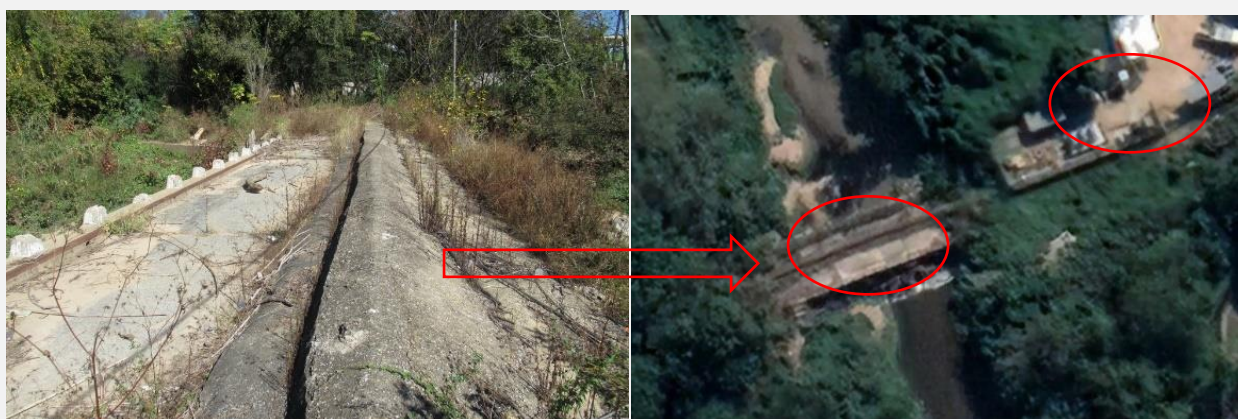
Figure 15. View of the old concrete road bridge
