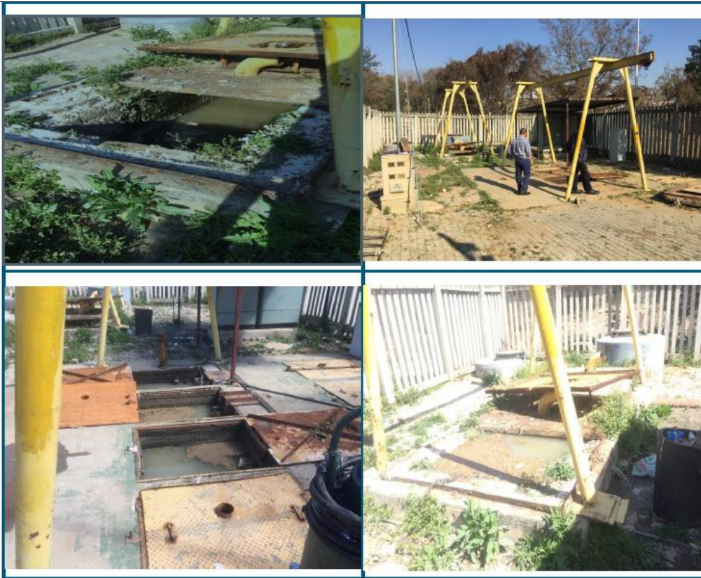
Figure 3: Status Quo of the Jukskei Pump Station Site
