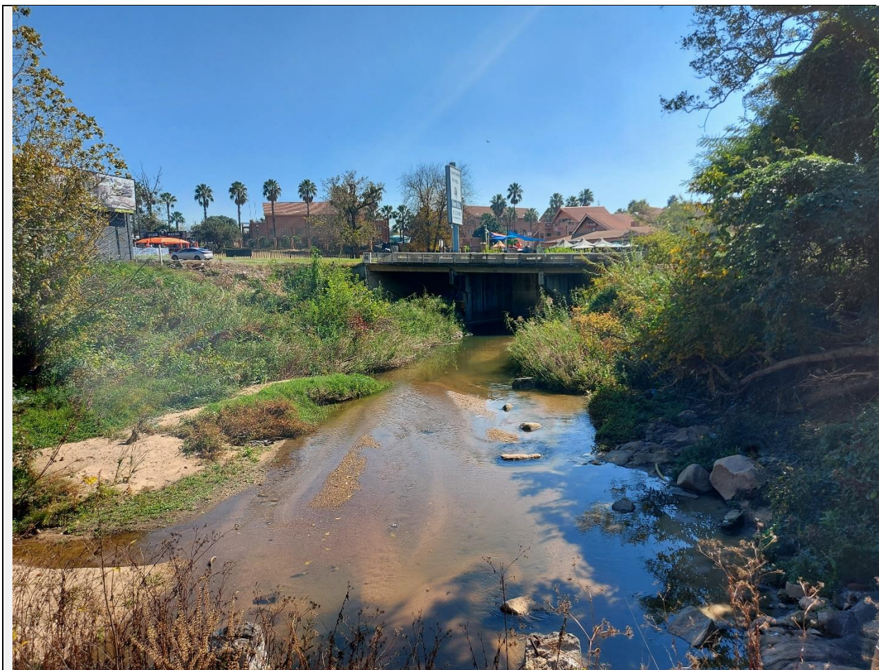
Figure 10: Alluvial deposits and large boulders visible in the marginal zone of the river.
