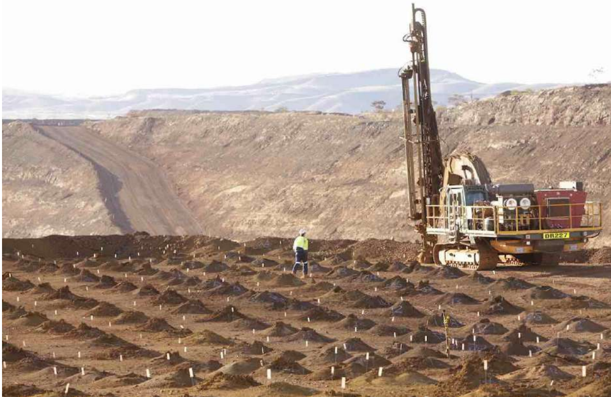
Figure 7: Blasting Design and Planning for Blasting
