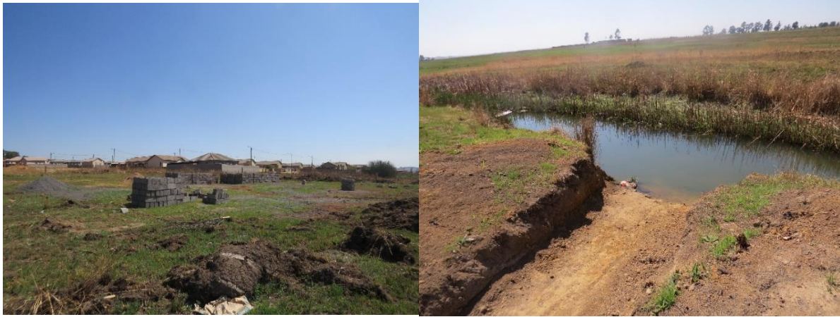
Figure 5.9: Images of impacts recorded within and surrounding the wetland areas including dumping, leaking sewerage and recent fires.
