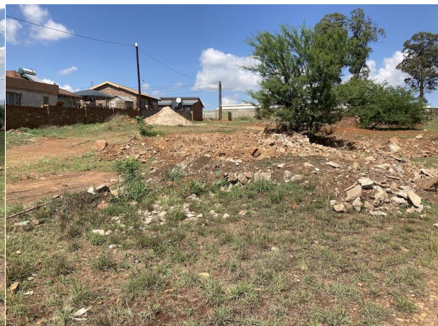
Figure 5.5b: Disturbed areas on site.
