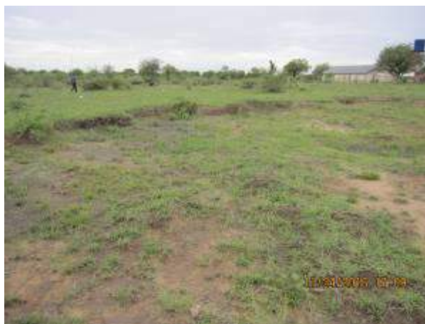
Harvesting of topsoil / excavations
