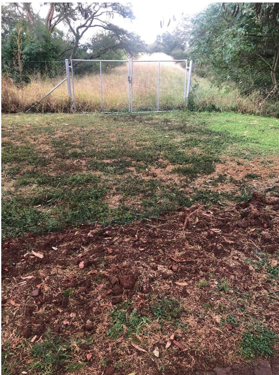
Figure 9. Current access gate to the right flank of the Ngodwana Club entrance leading onto the fuseplug embankment.
