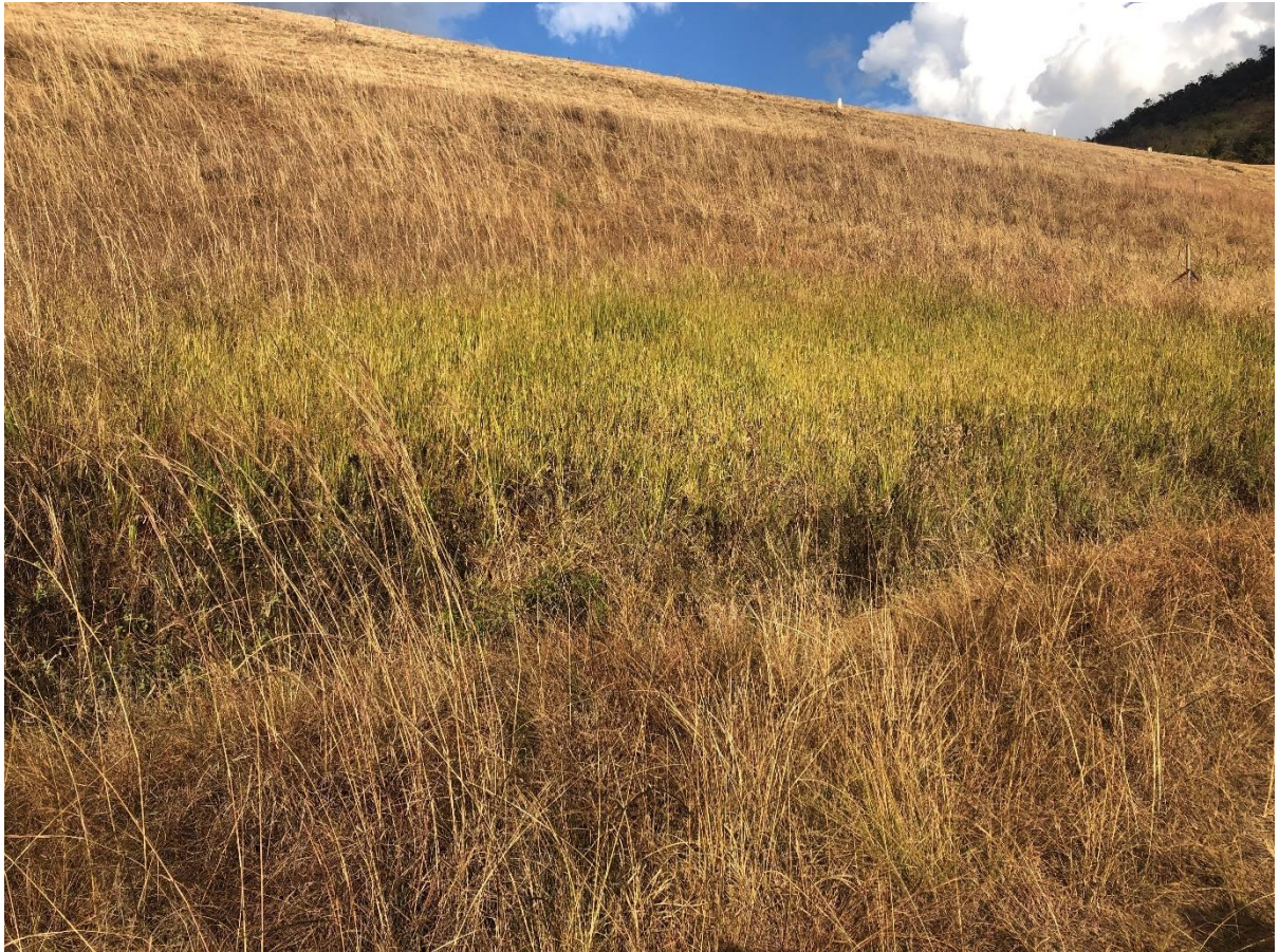
Photograph 2. The main embankment at the seepage “wet spot”.
