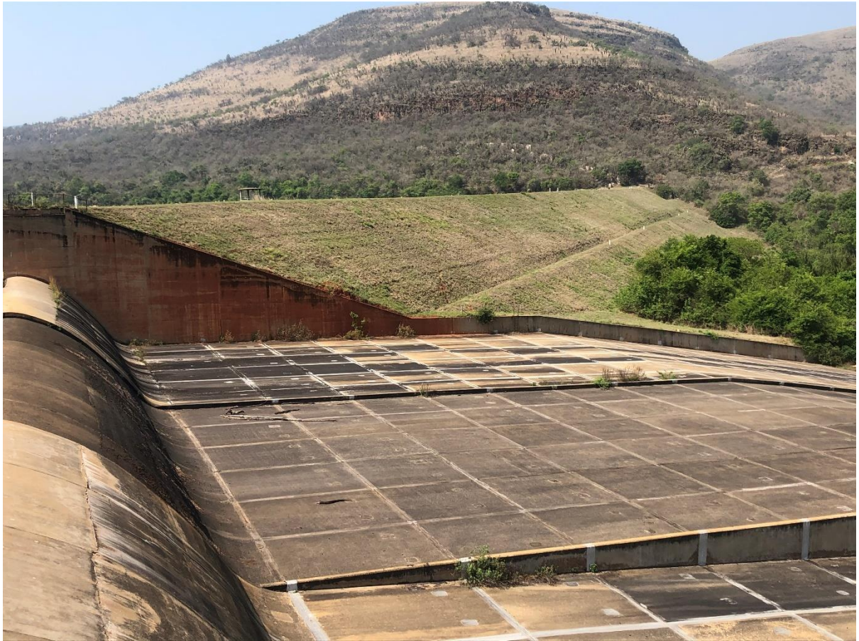
Photograph 4. The concrete spillway and main embankment.
