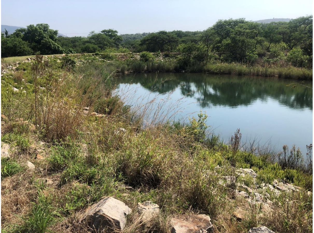
Photograph 3. The right flank (fuseplug) embankment.
