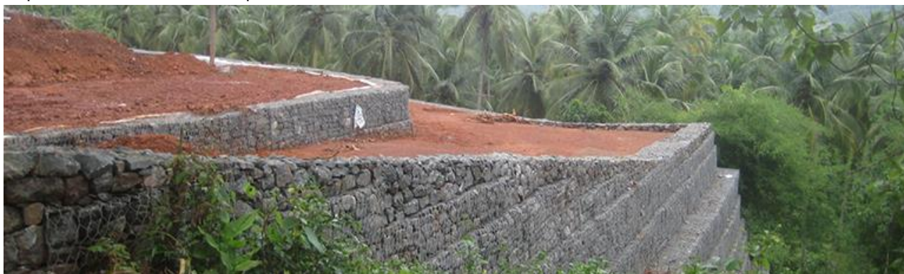
Figure 20: Gabion retaining wall.
