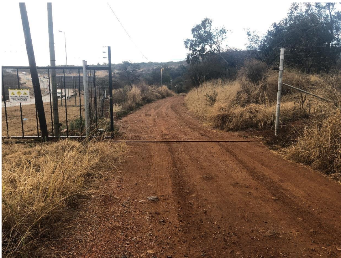
Figure 13. Gravel access road leading to SAPPI's Water Treatment Works (WTW).
