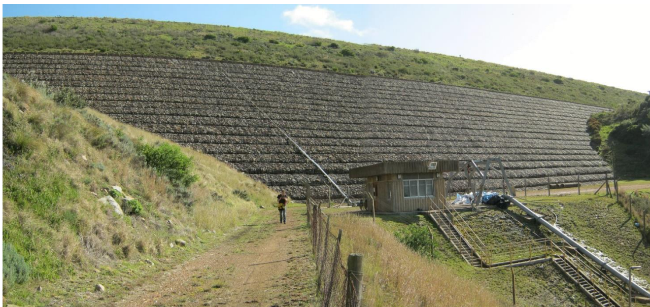
Figure 19. Reinforced rockfill used at Impofu Dam.
