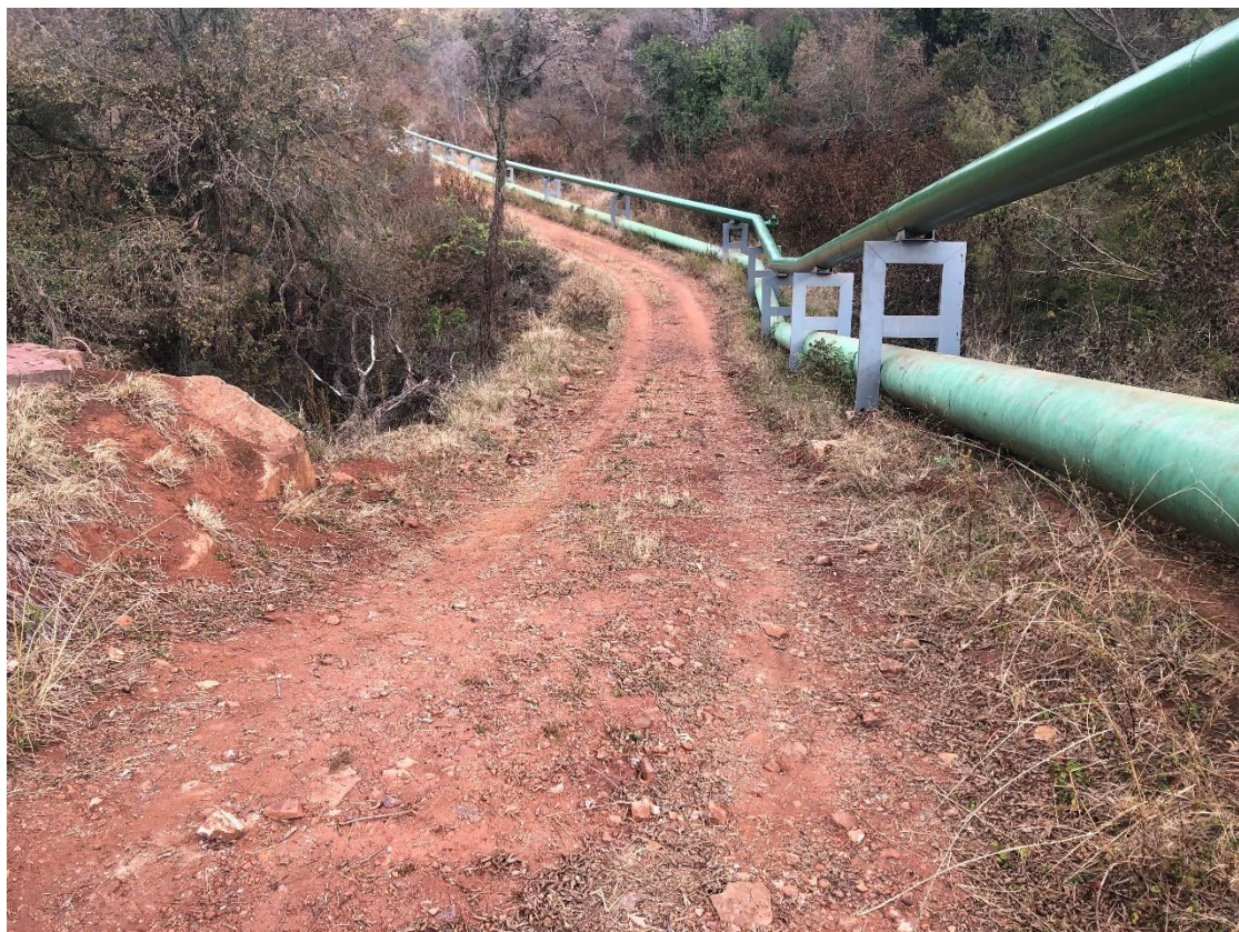
Figure 16. Existing gravel access road running from the WTW along the raw water pipeline to the main dam embankment.
