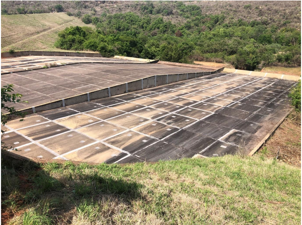
Photograph 5. The full extent of the concrete spillway interfacing with main embankment and right flank embankment.
