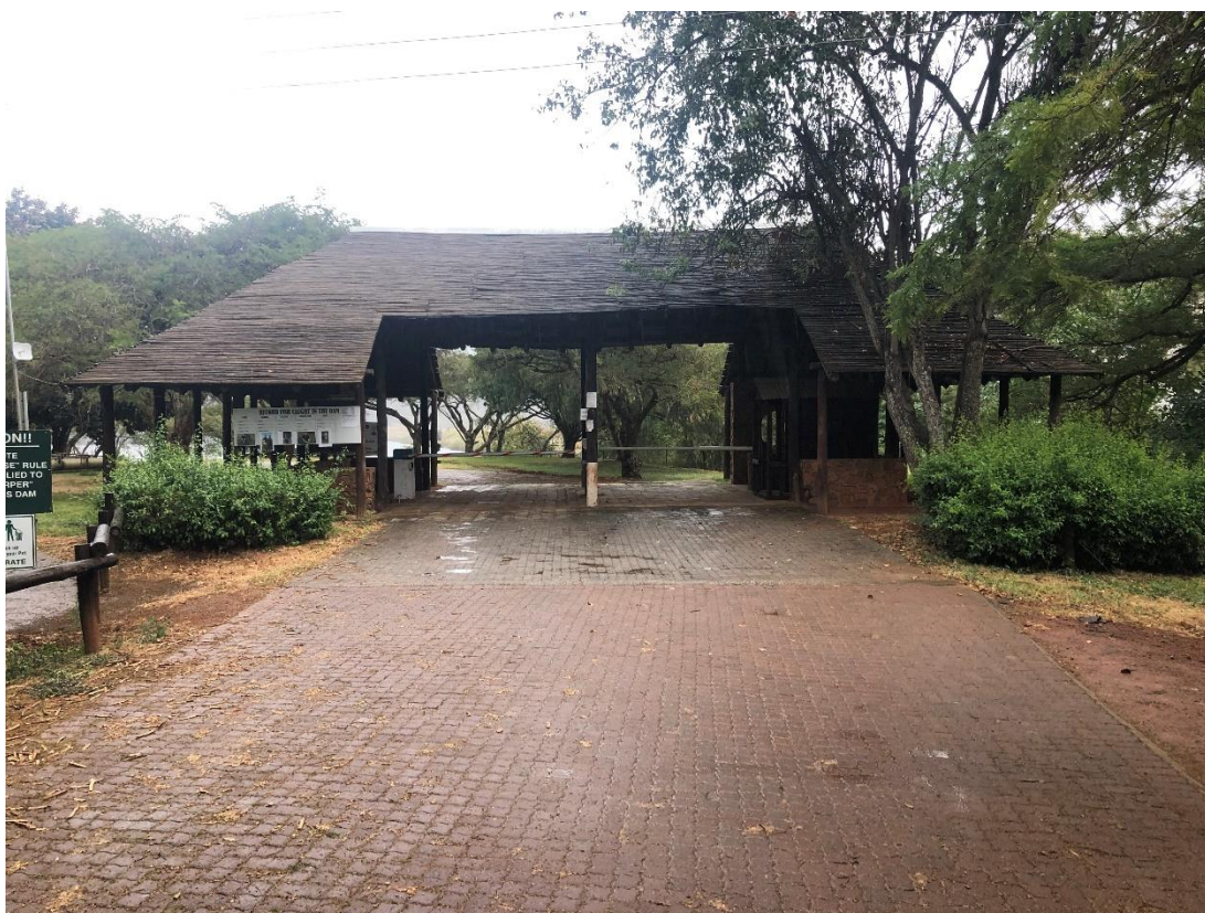
Figure 7. Current access road to the Ngodwana Club, for which an alternative road to the right will be required to allow for large haulage.
