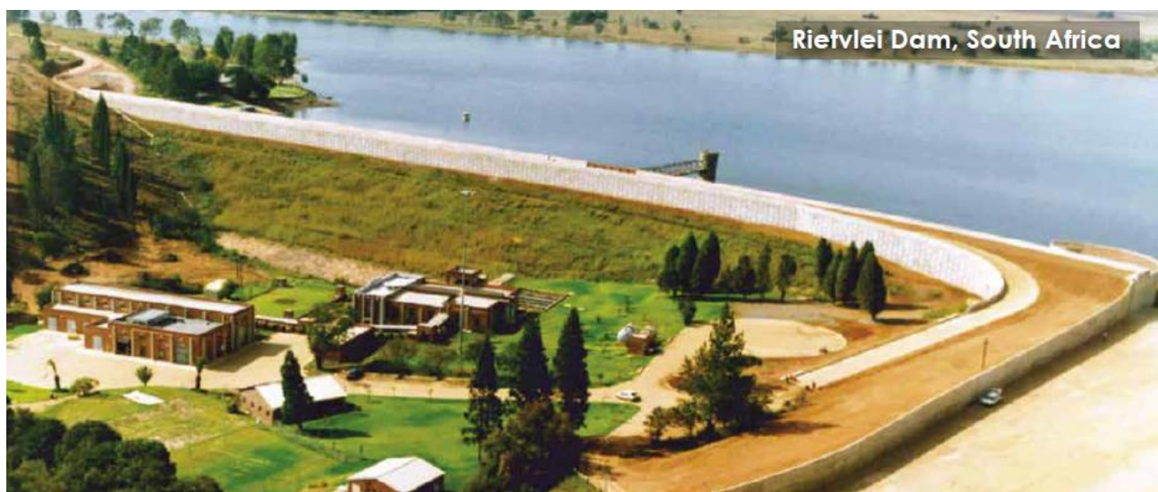
Figure 21: MSE raising of Rietvlei Dam.
