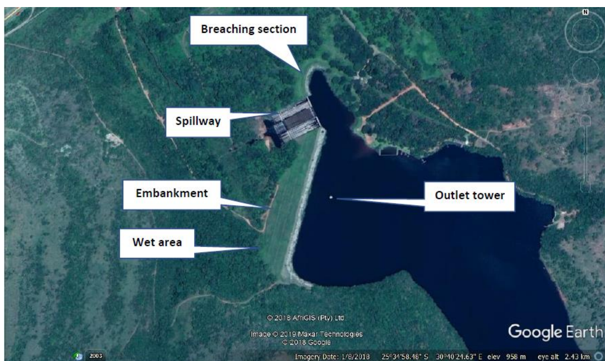
Figure22. Areas of concern on the Ngodwana Dam wall, for which remedial work will be required.
