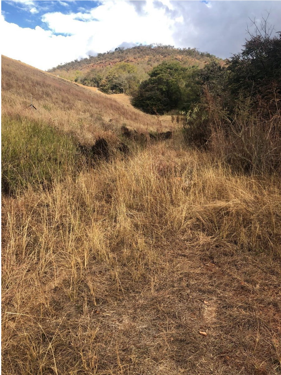
Photograph 1. Works Area 1: The main dam embankment south of the spillway.
