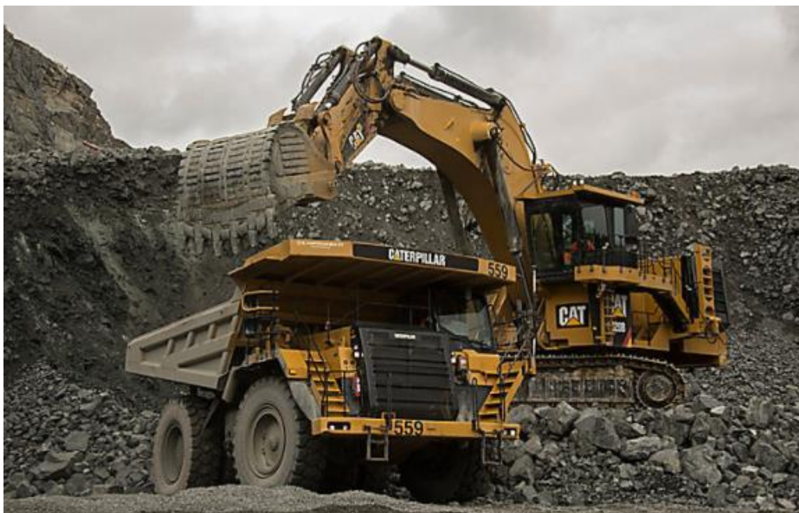
Figure 2: A typical truck and Backhoe Excavator operation (Internet Search)
