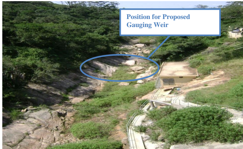
Figure 2: Proposed Site for EJ Smith Dam Gauging Weir
