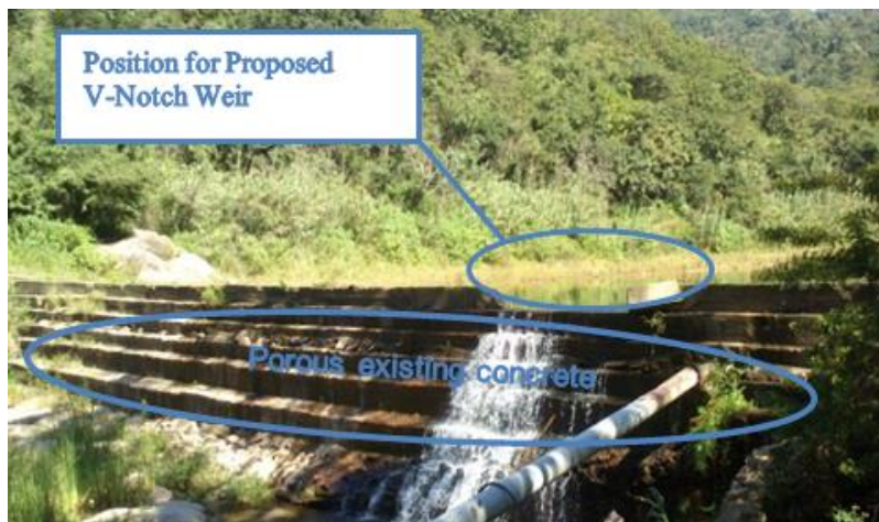
Figure 1: Existing Esperanza Raw Water Pump Station Abstraction Weir
