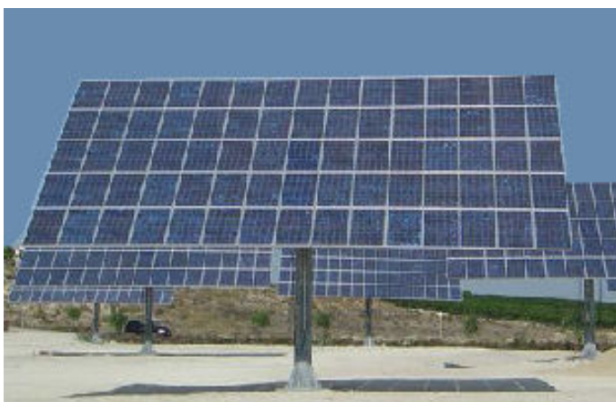
Figure 2.3: Illustration of a tracking photovoltaic panel
