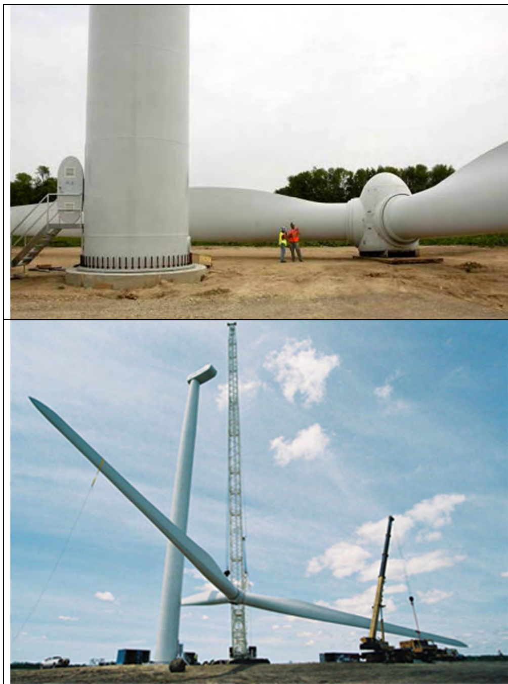
Figure 3-4: Wind turbines in the process of being erected 17
