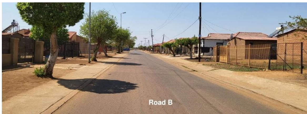
Figure 18: Existing Pedestrian Walkway along Road B (eastbound view along Road B)
