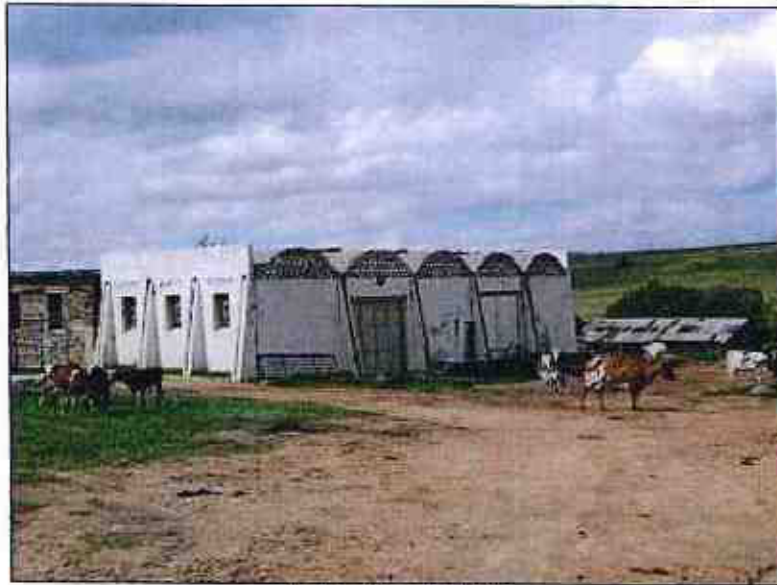
No 5e: Store building
