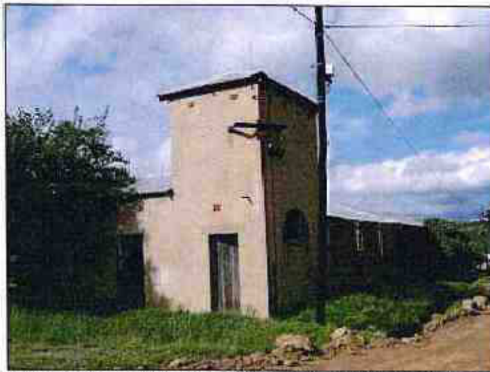
No 1d: Pumphouse and reservoir (to be preserved), with No 3c (left): Face brick store
