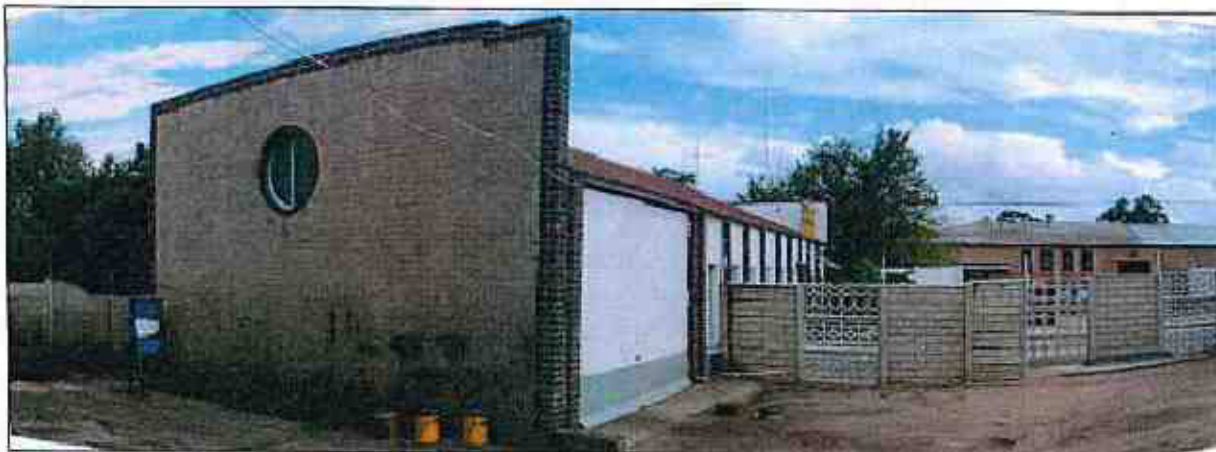
Buildings 5g (left) and 5f (right)
