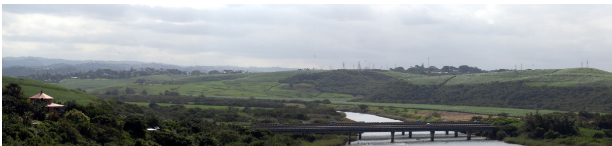
Figure 10-48 View north-west from LVP017, northern Illovo Beach, across the Lovu River floodplain. The Kingsburgh Major Substation is visible on the hills in the middle, as are the N2 and R102 bridges across the river.
