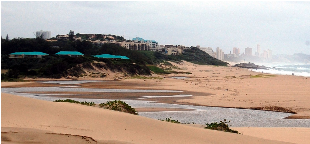
Figure 10-47 View from the beach at Illovo Beach towards the construction Jetty site. The Pump Station site is located behind the Boardwalk complex (turquoise roofs).
