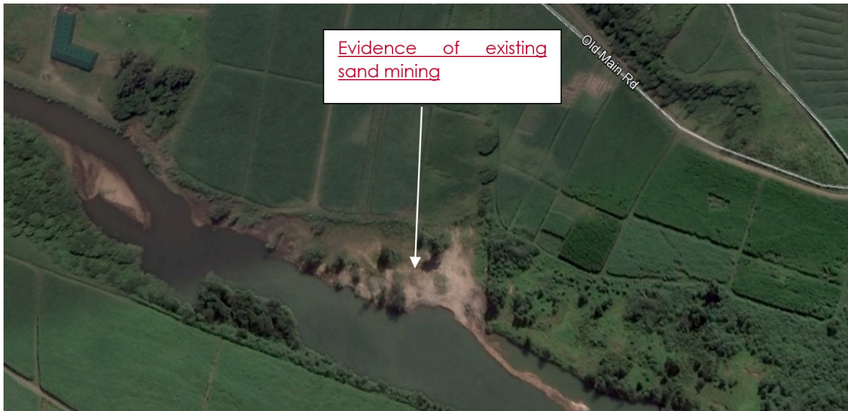
Figure 7.1b Evidence of sand mining along the northern bank of the Lovu River
