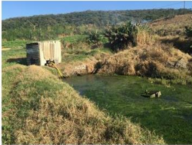
Photo E Excavated storage pond and pumped irrigation system in area just downslope of M4
