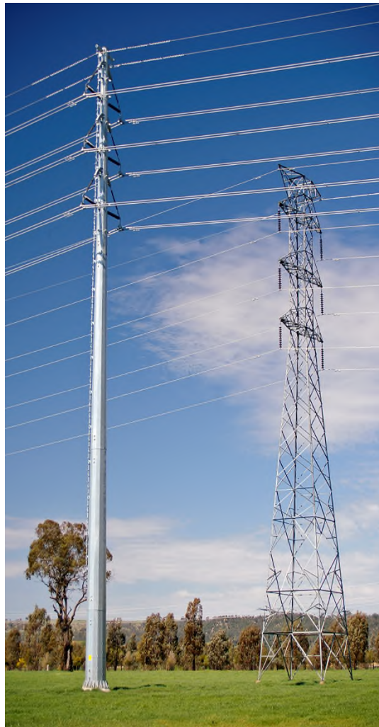
Figure 3.5: Examples of Monopole versus Lattice Tower designs
