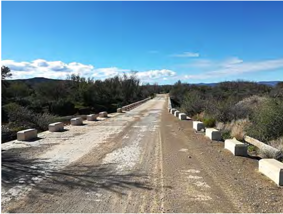
Figure 13: Narrow bridge on DR02249
