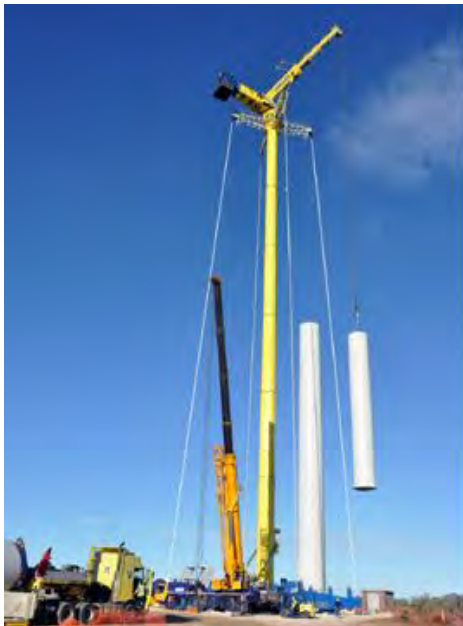
Figure 7: Cranes at work
